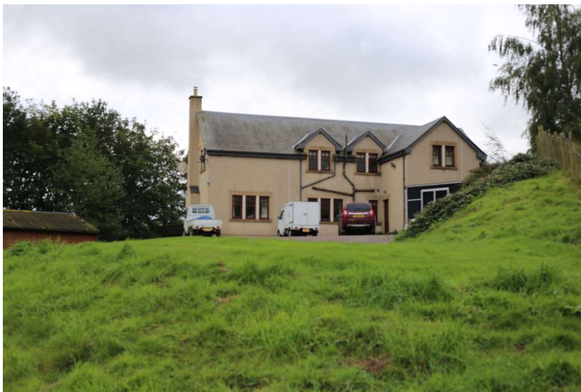
Image showing the rear aspect of Soonhope House which faces towards the proposed development
