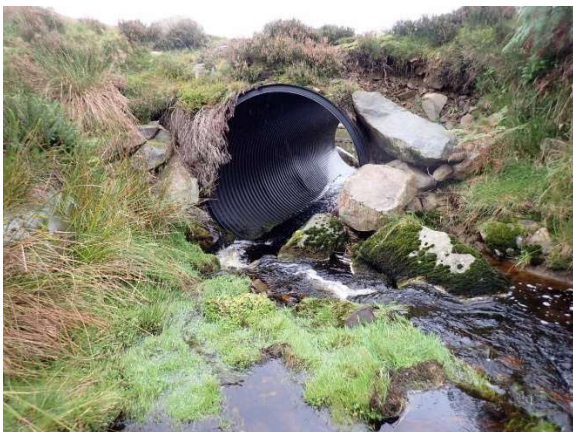
Plate 9: T10: Culvert
