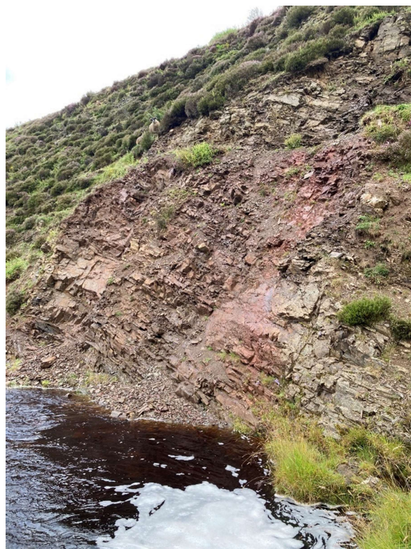
Photograph 10. T6 survey location: Bank erosion
